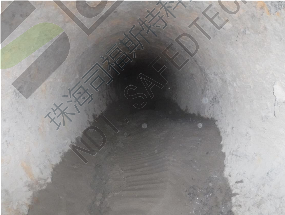
Photo shows the area with significant sediment buildup. This area is close to the condenser on the outlet side of the system.
