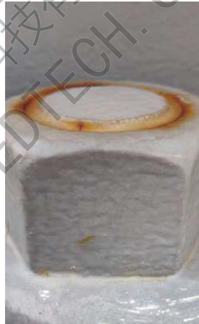
Lack of thread engagement on bolt at flange
