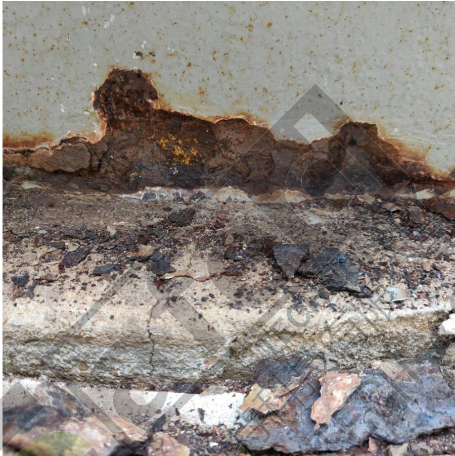
Coating Failure where Circulating Water Line comes out of the ground
