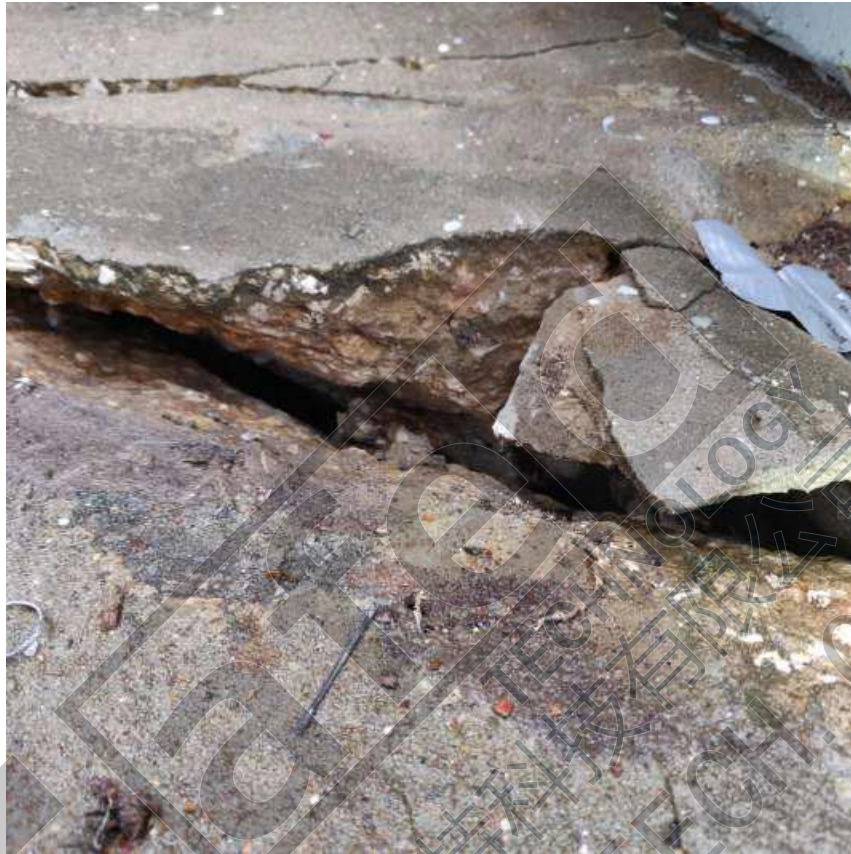
Cement base disintegration where Discharge pipe comes out of ground on Condenser side
